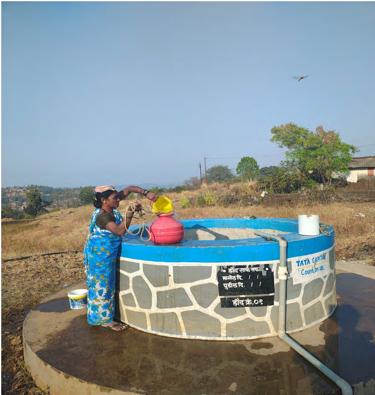
JalAadhar-Water Access intervention site-Mokhada | Source: Deloitte
