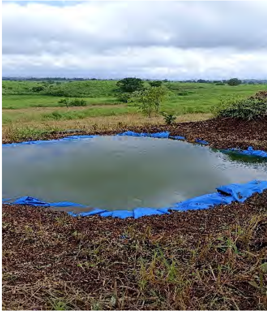
Image 4: HDPE sheet lined houth on line 1, Poshera
